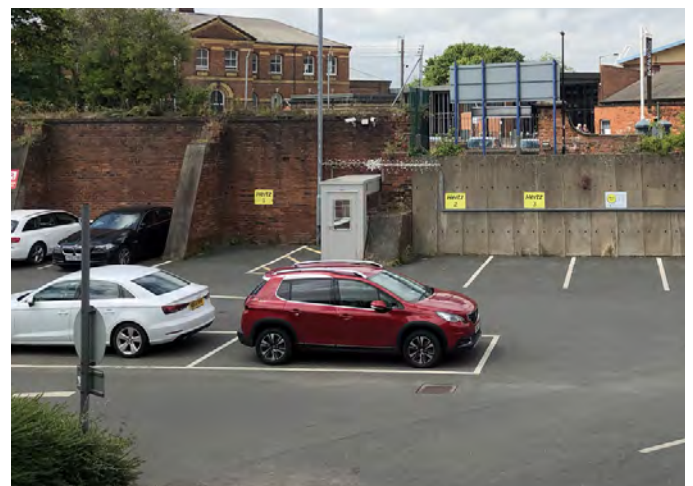
Fig.265 East face of the Coal Drops with the National Railway Museum beyond
