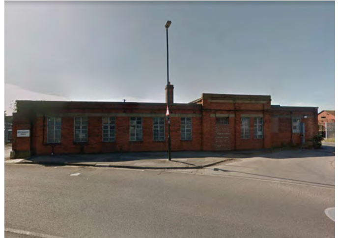
Fig.260 1930s building seen from Leeman Road
