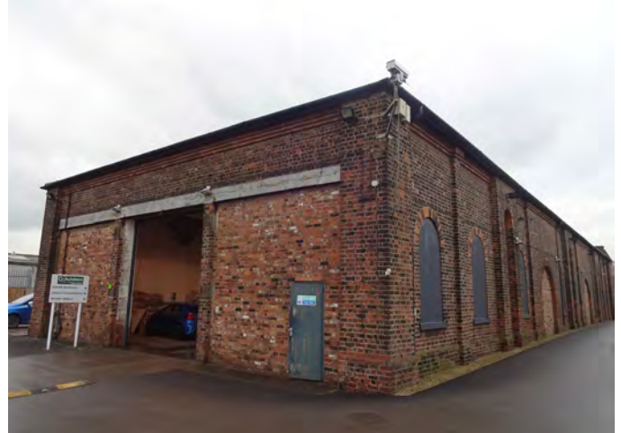
Fig.252 Albion Iron Foundry shop - main building - east facade
