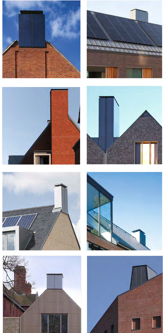
Fig.321 Examples of contemporary chimneys
