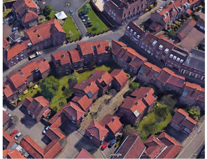
Fig.291 Small scale roofs to houses on St Andrewgate ✔️
