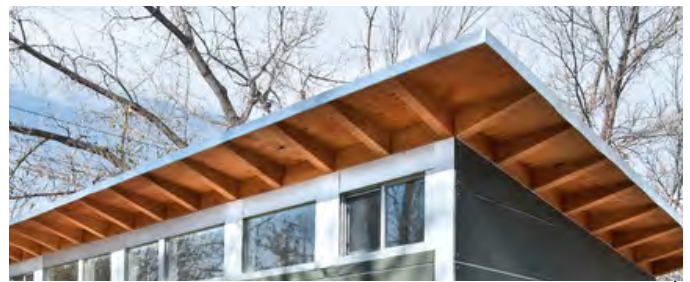
Fig.310 Example of a contemporary eaves detail
