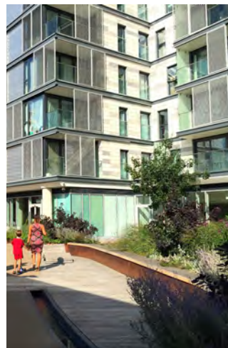
Fig.470 Inner courtyard panelled material ✓
