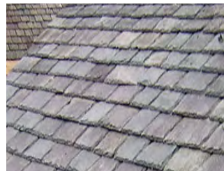
Fig.299 Lake District slates
