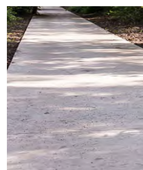
In-situ concrete with exposed aggregate
