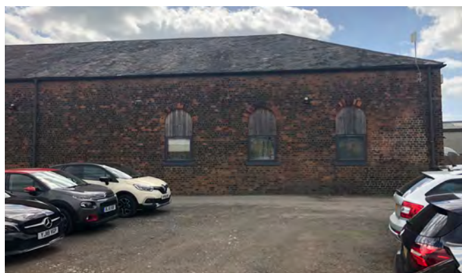
Fig.257 'Engine Shed' north facade east facade
