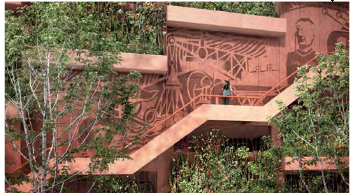
Fig.435 Car park with active facade
