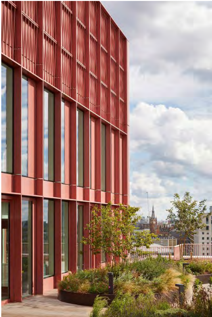
Fig.413 R7 Kings Cross office building, London Contemporary commercial buildings
