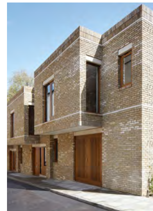
Fig.346 Example of contemporary jettied floors
