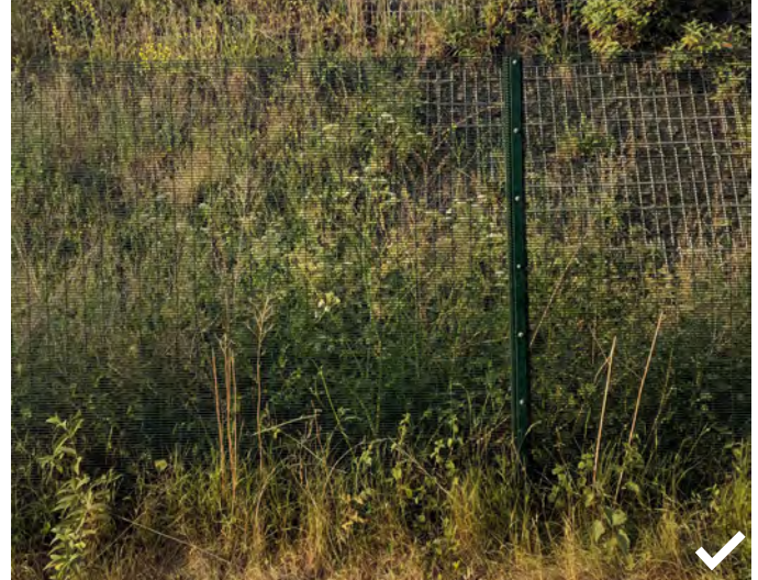
Fig.381 Green mesh blends into landscape. Fence to railway, Millwall
