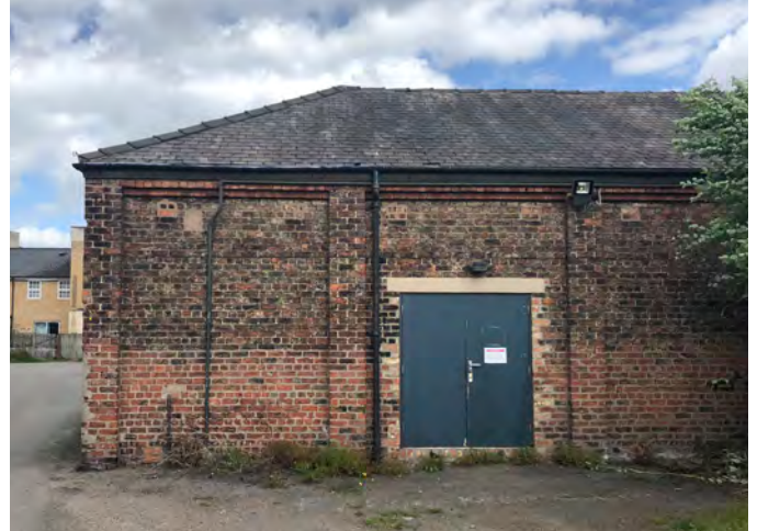
Fig.242 Existing railway shed in the Albion Foundry area
