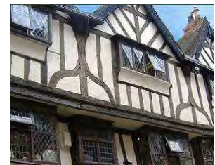
A historic jettied floor in York
