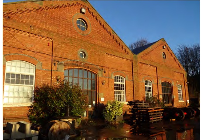
Fig.270 Carriage works stores and office, also known as Alliance House
