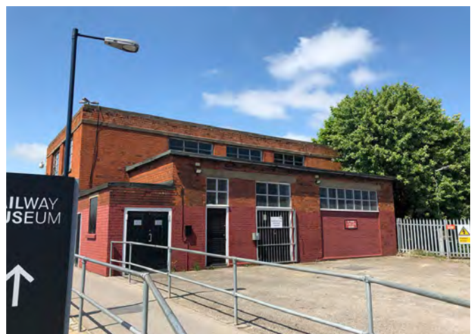
Fig.269 Generator building seen from the east
