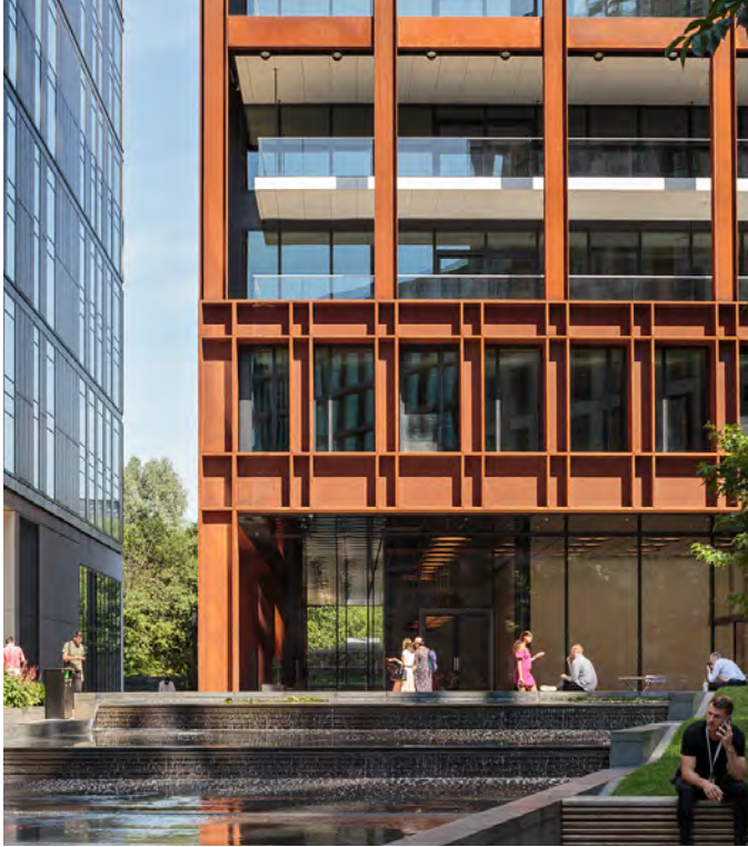
Fig.546 St Pancras Square, Kings Cross, London
