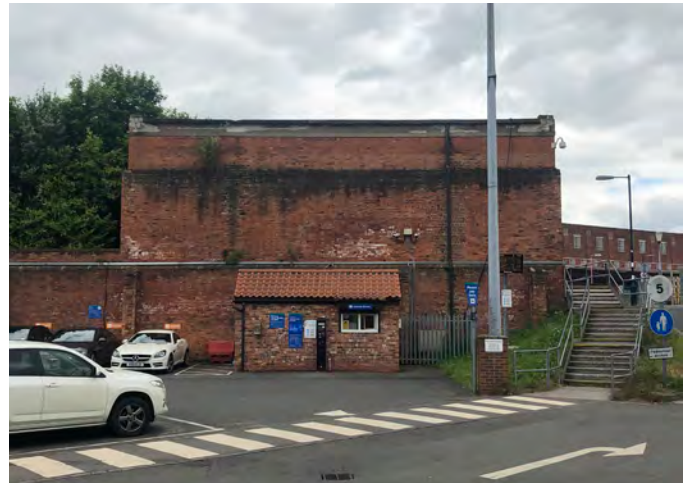
Fig.268 Generator building seen from the west
