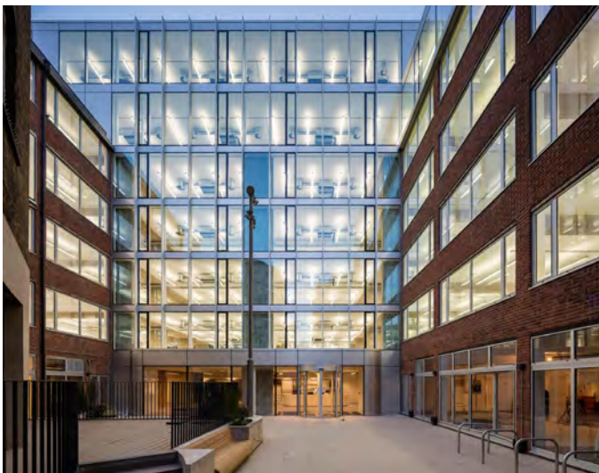
Fig.424 Fully glazed wall, Sutton Yard, Islington London
