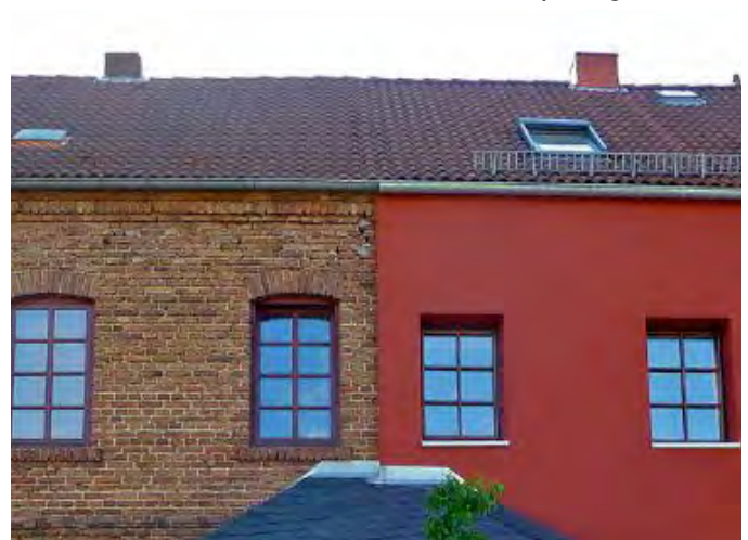
Fig.245 Exterior insulation covering brick details on historic building in Germany
