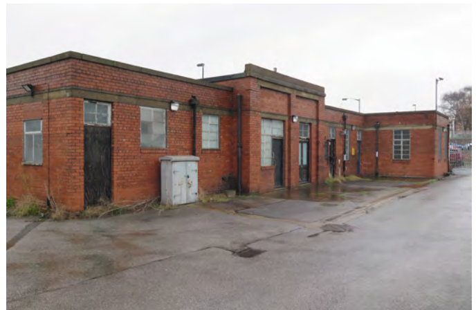
Fig.261 South elevation of 1930s Leeman Road building
