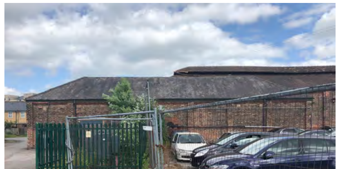
Fig.254 Albion Iron Foundry shop - parallel brick shed - west facade
