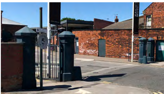
4 Gate Piers (Grade II listed)
