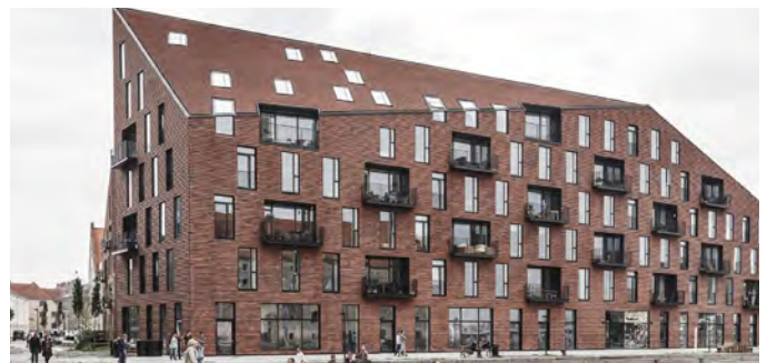
Fig.455 Example of a facade composition not suited to York Central. Though contemporary and well detailed, the uninterrupted roofline, single plane of walling, and regular balcony placement emphasise the monolithic quality of the block.
