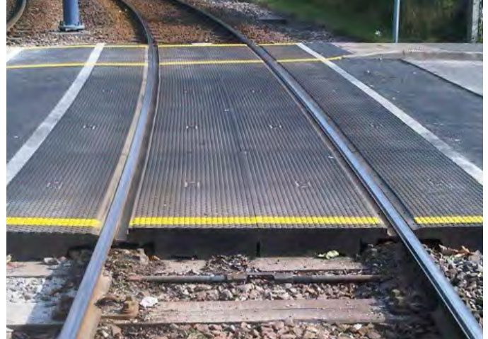
Fig.216 Embedded tracks within public highway
