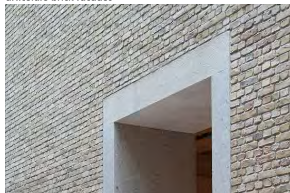
Example of a contrasting masonry material used to frame openings in brick walling
