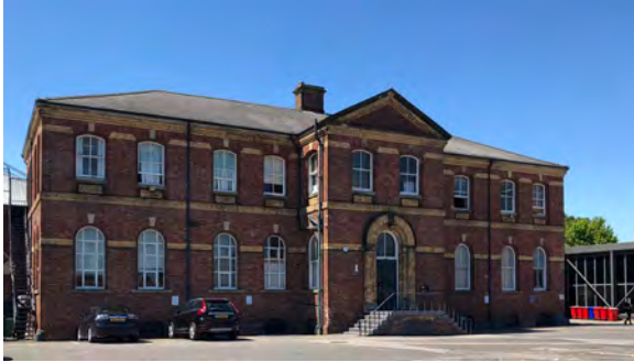
1 Former Goods Station (Grade II listed)
