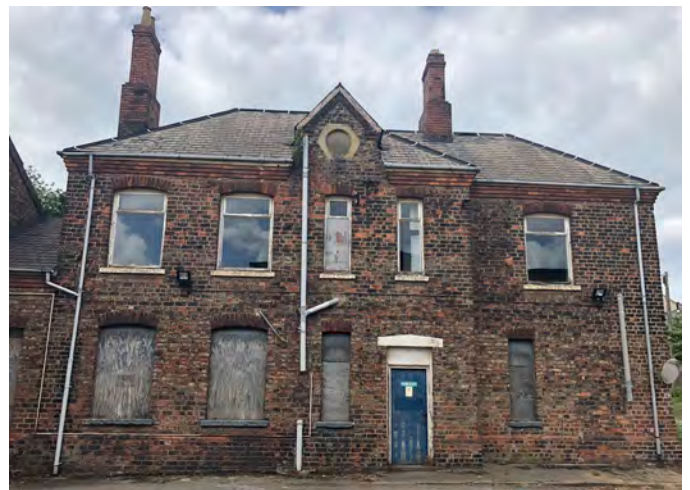
4 Smith's Shop Office
