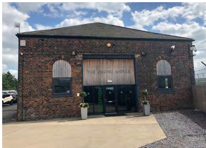
Fig.256 'Engine Shed' north facade
