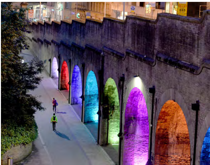
Fig.67 Illuminated arches (Saint Blaise Square, Bradford Council)
