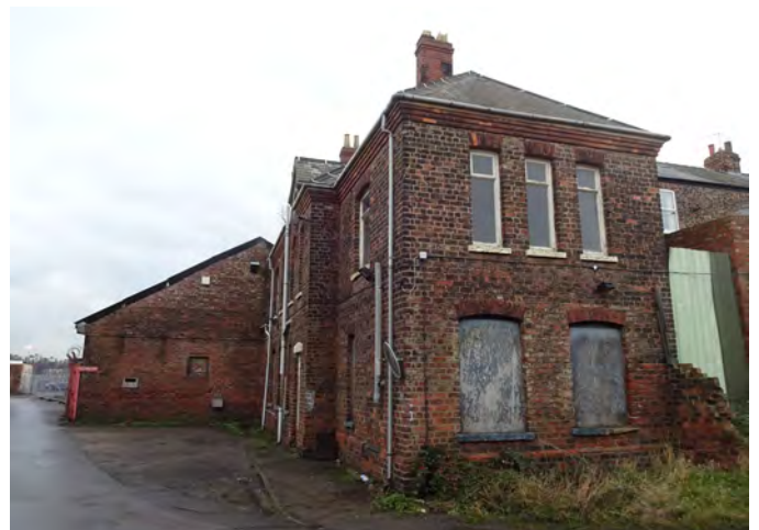
Fig.259 East frontage of Smith's Shop Office
