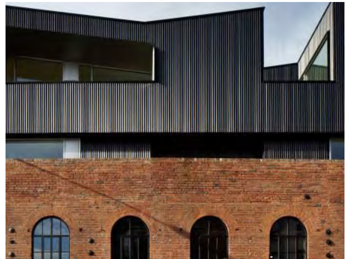
Fig.425 Metal sheeting, Shoreham Street, Sheffield
