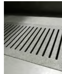
Bespoke channel drain made of stone
