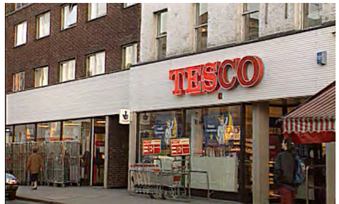
Fig.356 Shopfront fascia dominates building
