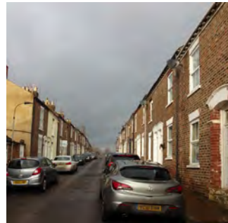
Fig.484 Railway worker housing on Carleton Street
