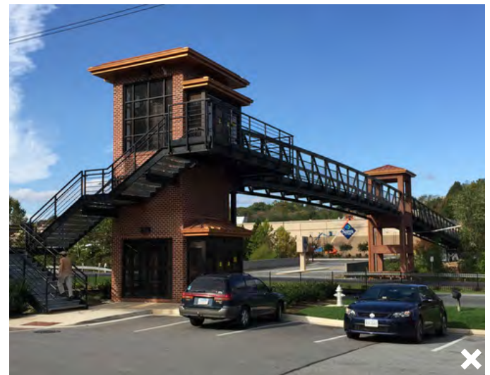
Fig.93 Example of inappropriate pedestrian crossing
