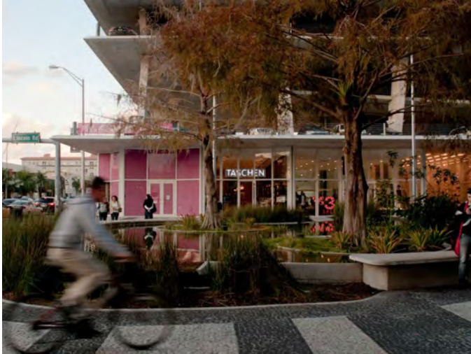
Fig.566 Lincoln Road, Miami Beach open car park structure can be used for other activities
