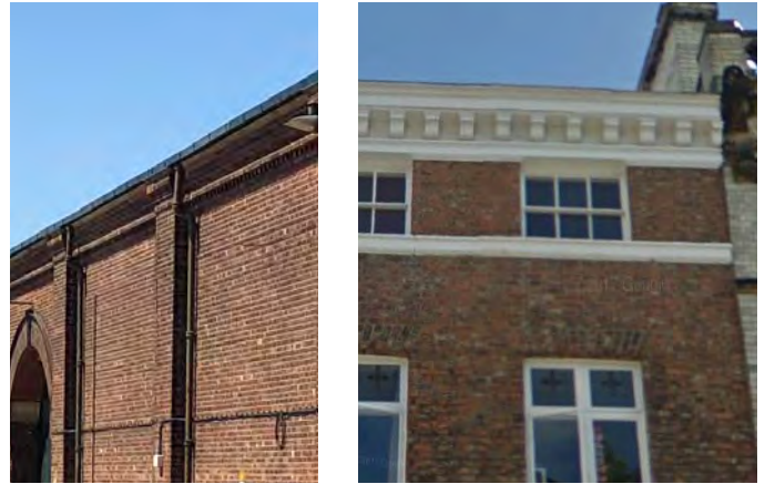
Fig.309 Examples of the many different existing eaves details in York
